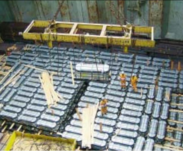
LOADING OF STEEL IN BRAZIL.
