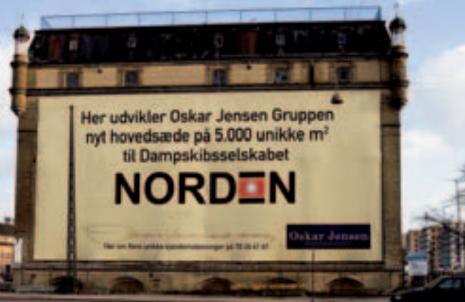
THE COMPREHENSIVE CONVERSION IS WELL UNDER WAY.
